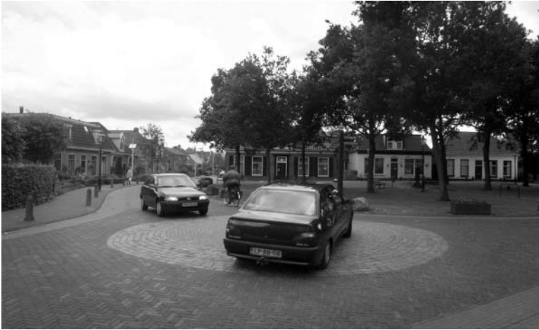
Figure 5. Makkinga, Friesland. All traffic signs, signals and markings removed. (Photo: Andrew Burmann)
